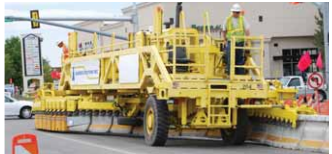
2 T.Y. Lin International, Evaluation of Moveable Barrier in Construction Work Zones
