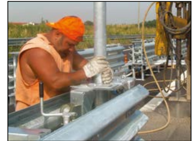
Figure 4 - Inserted Anchoring Picket
