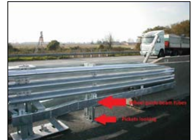
Figure 9 - Pickets looking and wheel guide beam tubes
