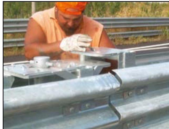
Figure 6 - Modules connected by Picket
