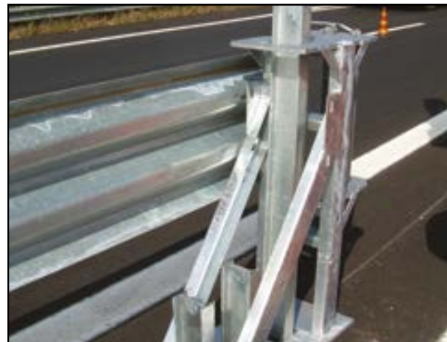
Figure 7 - Backup supports positioning
