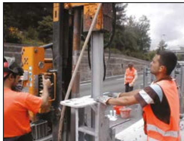
Figure 8 - Pickets insertion
