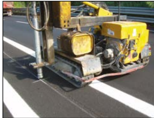
Figure 1 - Sleeve's insertion
