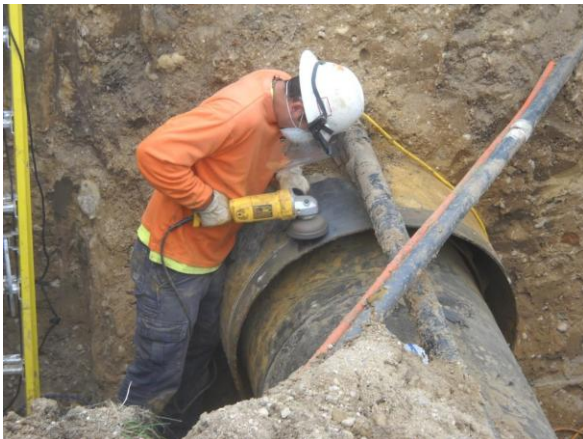
Figure 1: Cleaning the casing and pipe
