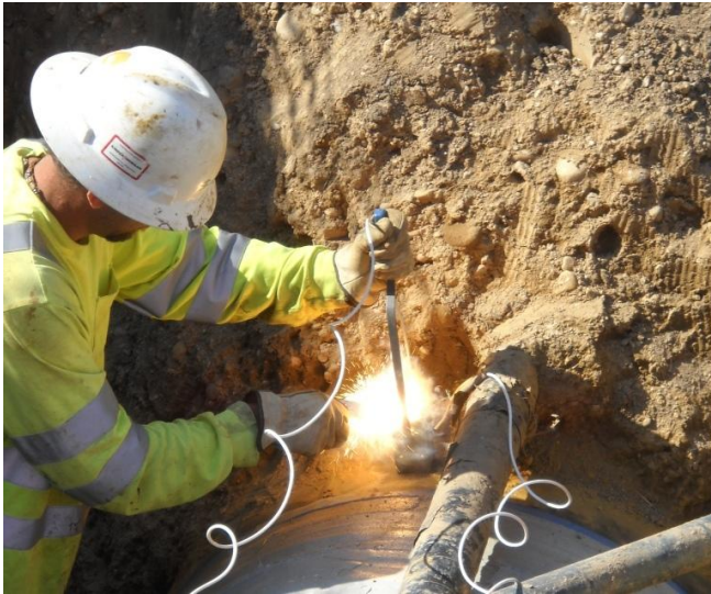
Figure 5: Welding leads to the casing.
