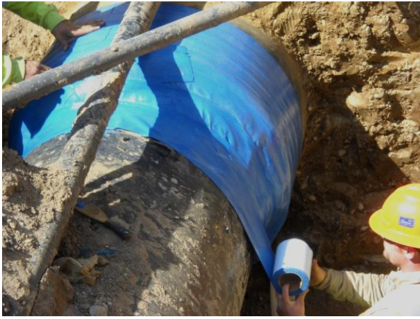
Figure 3: Adhesive wrapping applied over seal. Figure 4: Hardening overwrap applied.
