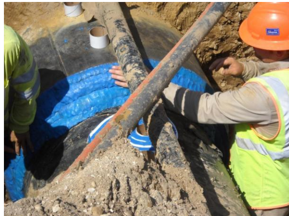
Figure 2: Sealing compound is installed between carrier pipe and casing.
