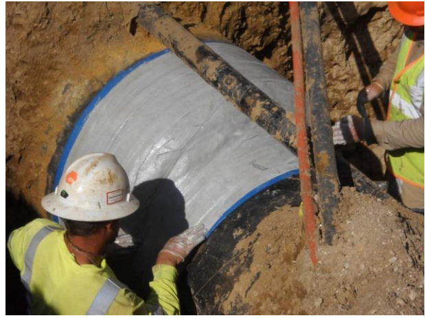
Figure 3: Adhesive wrapping applied over seal. Figure 4: Hardening overwrap applied.
