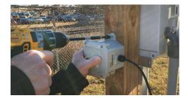
Step 5: Secure the unit to a post or wall using lag bolts or self-tapping hex head screws (not included).
