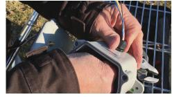
Step 3: Thread cabling through cord plug in the side of the unit.
