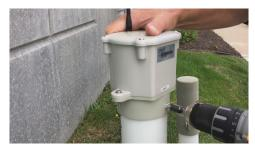
Step 3: For top mount installation insert excess wire inside of post and place top of post adapter in position on the post. Use self-tapping screws (not included) to secure the Tracker LT unit to the post. For side mount installation secure cable to post or wall to allow for strain relief of the connections.
