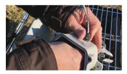
Step 7: Cut the cable to the proper length and connect the wires per the wiring diagram.
