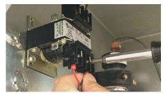
Step 6: Wire the input of the Transformer with a 120V or 240V supply from the commercial power input for the rectifier. Then connect the power wires from the Scout unit to the Transformer output.
