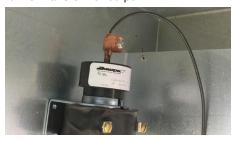
Step 7: Remove the Pipe wire from the negative output of the rectifier and connect it into the bottom of the mercury switch. Cut a length of same gauge wire to be connected from the top of the mercury switch to the negative output of the rectifier.
