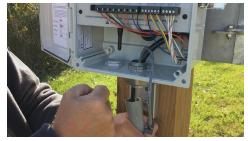
Step 4: Route the cables from inside the Scout unit through the conduit into the rectifier.
