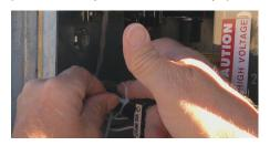
Step 9: Zip-tie AC detect probe to one leg of incoming AC to the rectifier.
