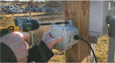
Step 5: Secure the unit to a post or wall using lag bolts or self-tapping hex head screws (not included).
