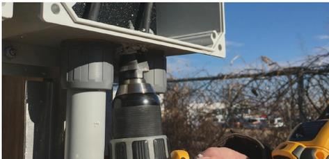
Step 6: If necessary, drill hole in junction box, install cord grip (not included), and route the cable into the junction box.
