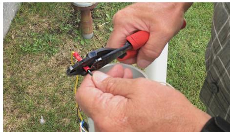
Step 2: Cut the cable to the proper length for the test site and connect the wires per the wiring diagram below (Brown, Yellow, & optional Blue/White wires). NOTE: Be sure to use electrical tape to insulate unused wires to eliminate possible shorts or errant grounding.
