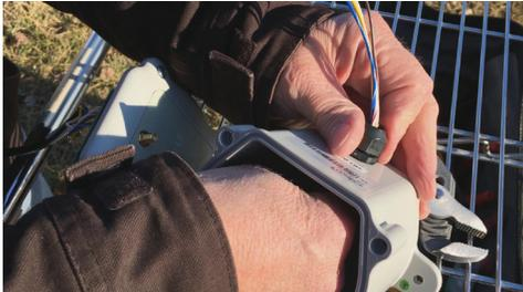
Step 7: Cut the cable to the proper length and connect the wires per the wiring diagram.
