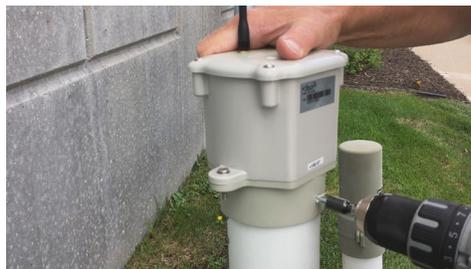
Step 3: **For top mount installation** insert excess wire inside of post and place top of post adapter in position on the post. Use self-tapping screws (not included) to secure the Tracker LT unit to the post. **For side mount installation** secure cable to post or wall to allow for strain relief of the connections.
