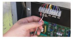
Step 8: Locate the Red, Black, White, and Green wires from the signal cable. Connect the Red wire to the Rectifier positive output and the Black wire to the Rectifier negative output using the ring or fork connectors provided. Connect the White wire to the Shunt positive output and the Green wire to the Shunt negative output with the fork connectors provided.
