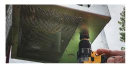
Step 3: Drill a 1-3/8" hole in the bottom of the rectifier using a 1-3/8" stepped bit. Install a 1" conduit connector in the hole. Cut a piece of 1" flexible conduit that will reach from the Scout unit to the bottom of the rectifier.
