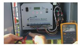
Step 12: Unplug the power plug from the Scout unit, turn on the rectifier power, and using a multimeter set for VAC, measure the voltage on the screws of the Scout power plug. The reading should be 12VAC to 14VAC. Plug in the power plug and turn the Scout unit switch on. Allow 5 – 10 minutes for the Scout unit to initialize and lock the GPS signal. Call Elecsys Customer Support, 913-825-6366, for help configuring the new unit on the Elecsys Website.
