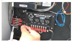
Step 2: Remove the power wires from the terminal block on the lower left of the WD2 enclosure.
