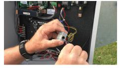
Step 5: Disconnect the wire from the bottom of the Mercury relay and remove the current sensor from around the wire. Reconnect the wire to the bottom of the relay. Disconnect the red and black wires from the body of the relay.
