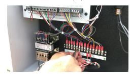
Step 10: Install all fork terminals from the signal cable in the appropriate screws of the Terminal Strip.
