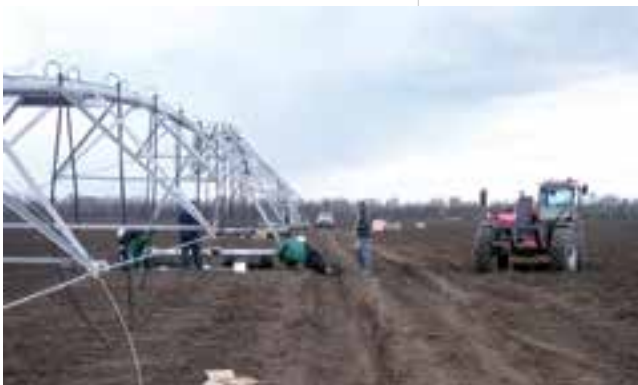
The Zimmatic® by Lindsay laterals and pivots were carefully designed not to contribute to soil compaction.
