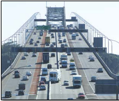
Moveable medians are the only barrier on the roadway
