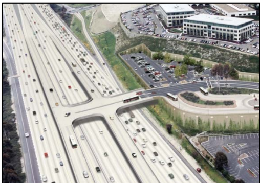
Direct access ramps for Express Lanes users and BRT
