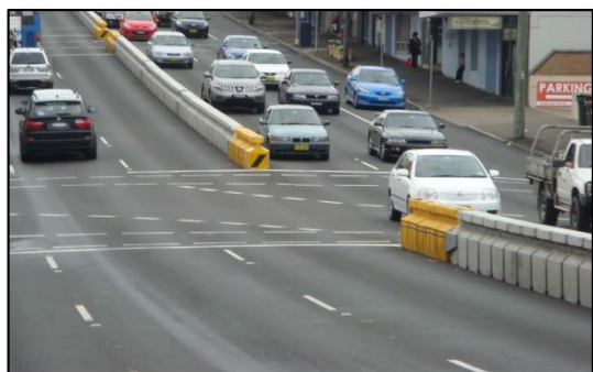
Sydney: Moveable barrier quickly reconfigures the roadway Sydney: BRT travel time and reliability goals were met on Day One
