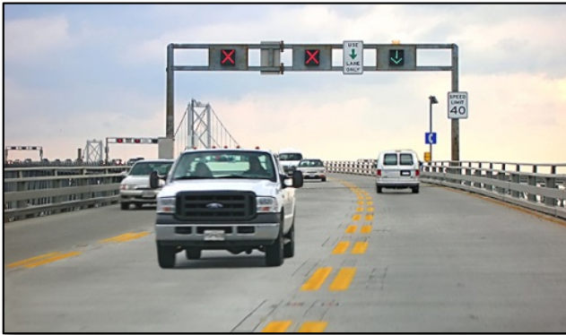
Lane shift using overhead lights and paint buffers
