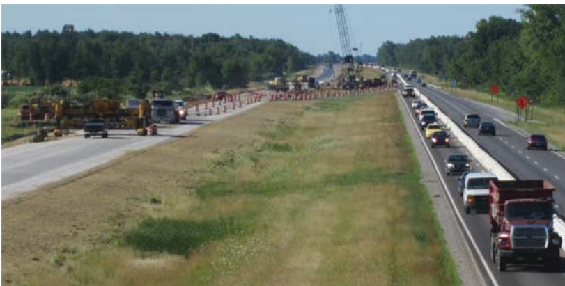
Traffic is crossed over and Moveable Barrier creates a 1/2, 2/1 configuration
