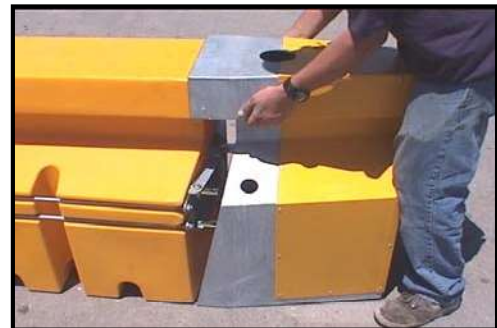
QMB Nose – Slide the corners over final element
