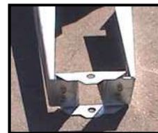
View of the pin end of the strap assembly after bolting up
