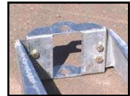
View of the pin end of the strap assembly after bolting up
