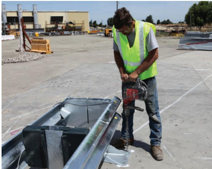
**Note: NOT ALL HOLES ARE REQUIRED FOR A CONCRETE INSTALLATION.** The holes identified with a notch are the required anchor points for a concrete installation. Refer to Appendix B, page 40.
