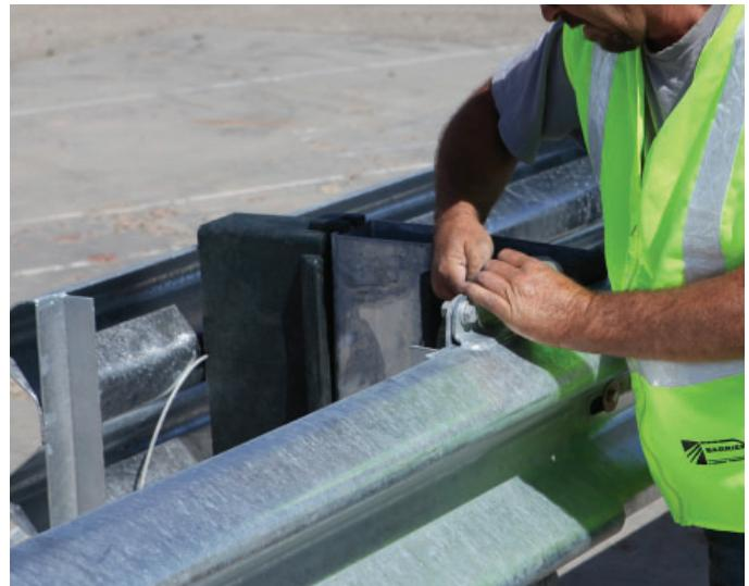
**Tip:** Assemble the M10 x 230mm bolt with washers and nuts and position the assembled bolts at each leg and the slider brace and M12 x 35mm bolts, washer and nuts at post THREE prior to positioning the panel in place so that the hardware and slider brace are easily assessable when ready to bolt on the panel and slider brace.
