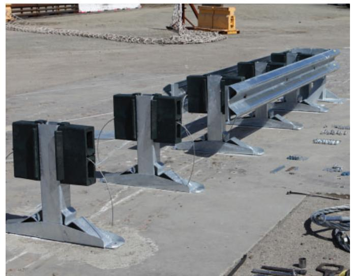
**Tip:** Assemble the M10 x 230mm bolts with washers and nuts. Position the assembled bolts at each leg and the shear bolts at the backstop prior to positioning the panel in place so that the hardware is easily assessable when ready to bolt on the panel.
