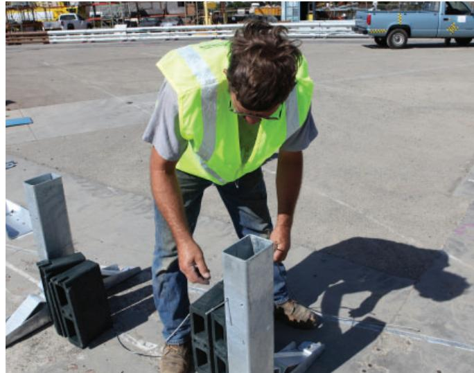
2b. Next, install two (2) blockouts on each post, one (1) on each side. At each post, guide the wire tether through the front hole of each blockout.
