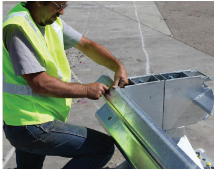
3b. The panel is now in place, finish by installing the remainder of the guardrail bolts and shear bolts to secure the panel to the backstop and the posts.
