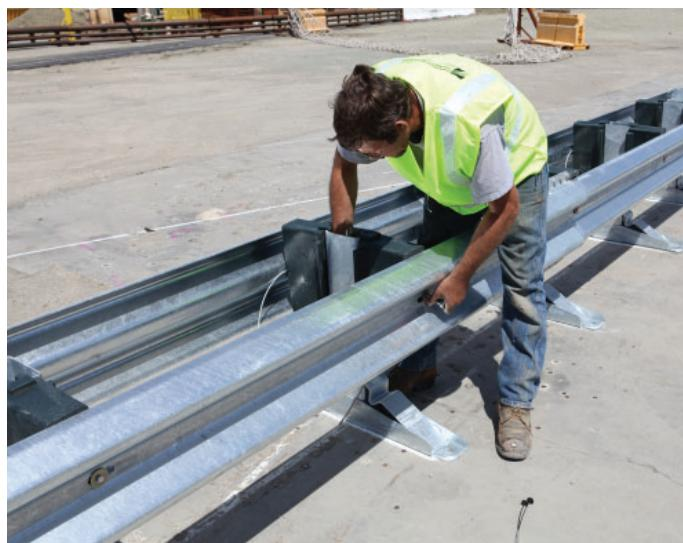
6d. Begin to drill all required holes for installation.
