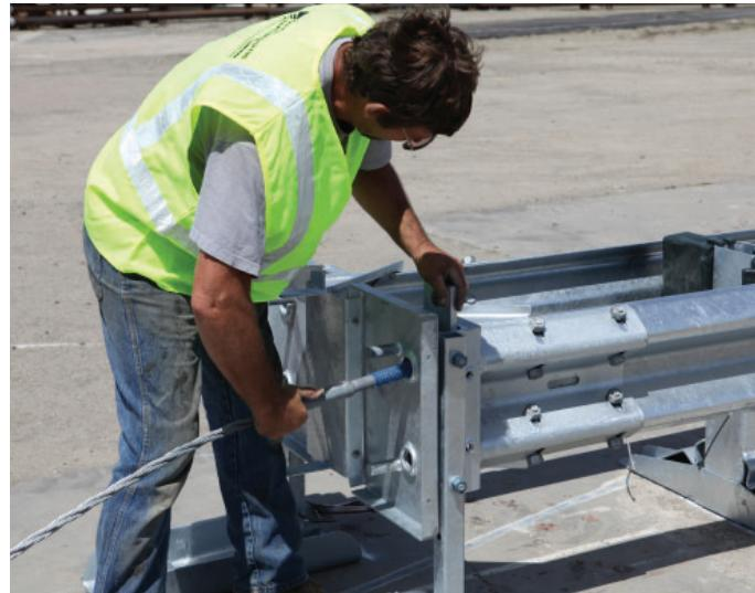
**Note:** If you removed a washer from the back end of the cable, do not re-install the washer. The washer may be discarded.
