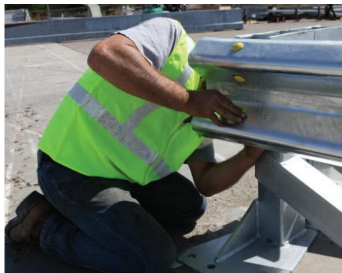
**Note:** When bolting on the panel at the posts, make sure that the wire tether does not get stuck between the blockout and the panel. Make sure that the wire tether is positioned inside the notch on the blockout which allows the wire tether to move freely once the panel is installed.
