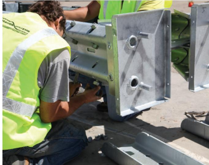
5g. Once the full head unit is installed, use the M20 x 65mm bolts with shoulder to secure the upper head support to the head unit. Next, install the lower head support using the M20 x 60mm bolts.
