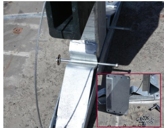
**Note:** The only hardware that should be tightened at this point is Slider Brace hardware. ALL OTHER HARDWARE WILL BE TIGHTENED AT A LATER STEP.
