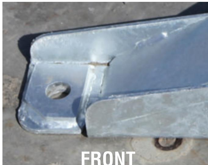
**Note:** Special attention must be taken when positioning the posts. The bottom plate of the posts is bent up on the back and front of the post. The front of the post has a shorter bend and the anchor holes are exposed. This side should be facing the front of the system.
