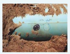
Undetected aggressive AC interference can cause serious corrosion in buried pipelines.
