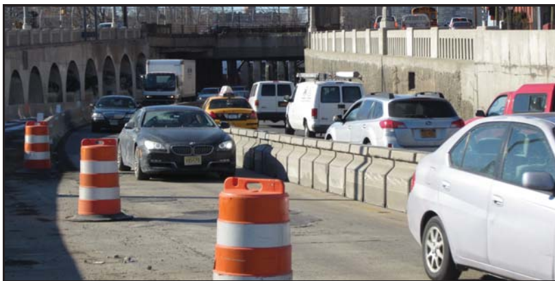
Moveable Barrier is used in a 1/2, 2/1 configuration to mitigate congestion
