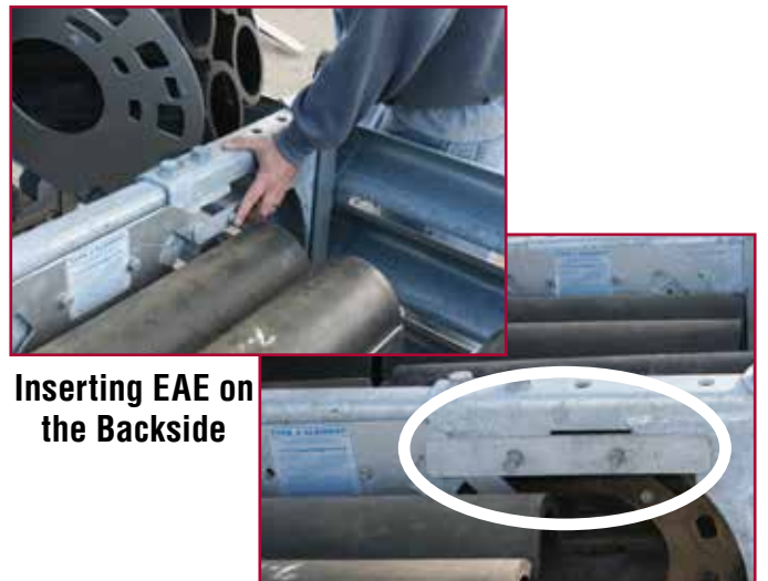
EAE Secured with Mounting Bracket
