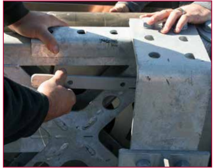
Using Mounting Bar to Attach EAEs
