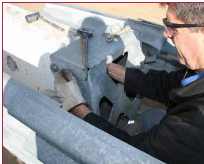
Removing Bolts from Flush Mount Backstop
