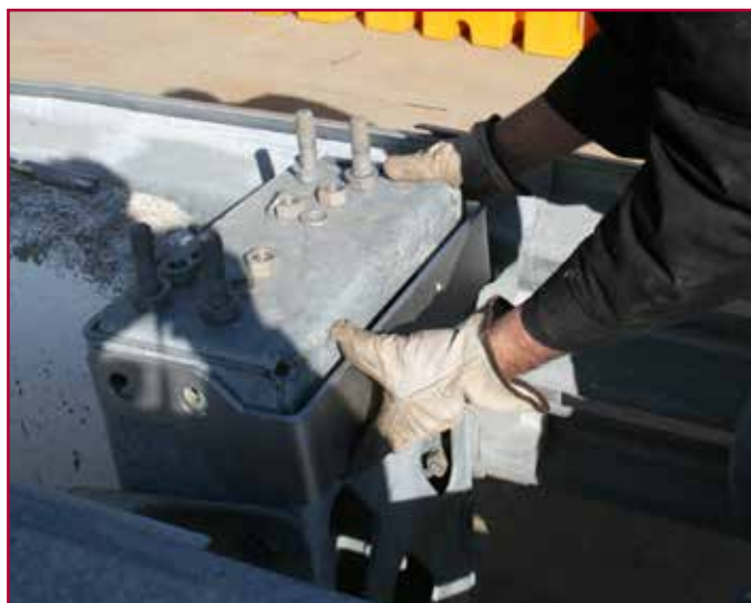
Sliding Bracket Over Backstop
