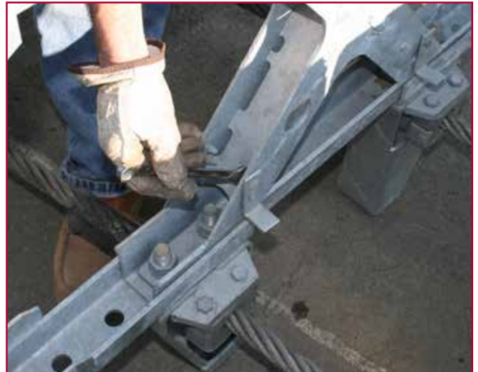
Removing EAC Locator Tabs
