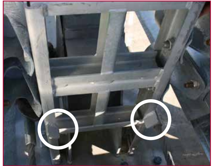
Tabs at the Bottom of Compact Backstop
