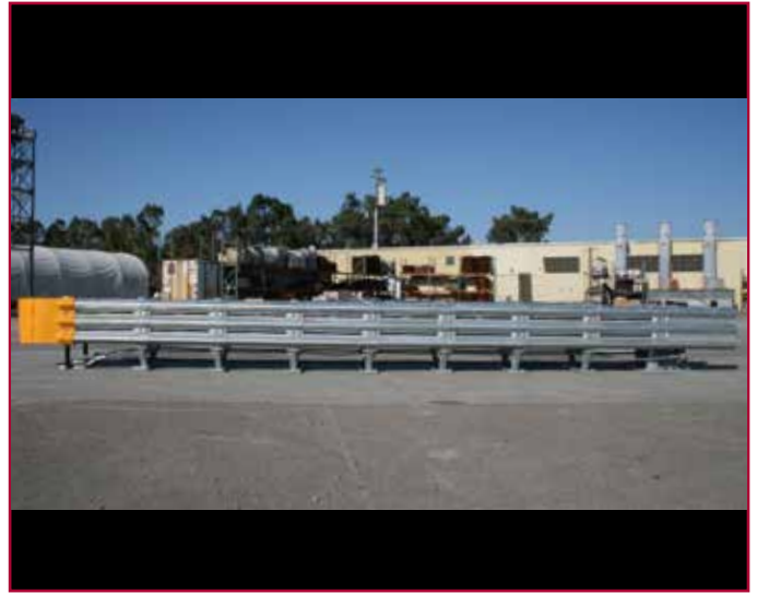
System Fully Extended and Panels Properly Lapped
