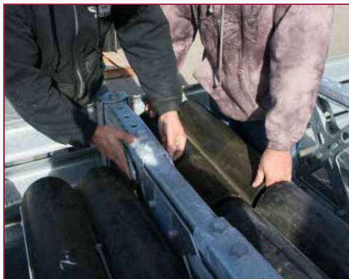
Securing EAEs Using Mounting Bracket
