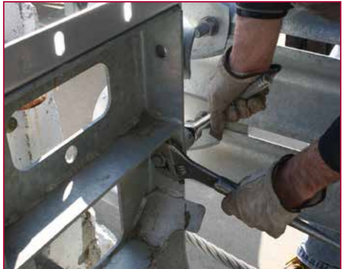
Securing PCB Bracket
