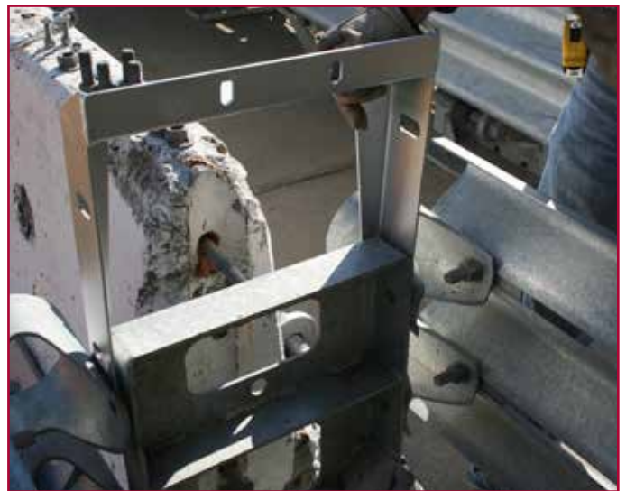
Sliding PCB Bracket over Backstop
