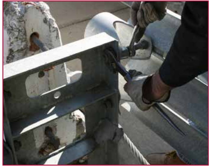
Removing Bolts from Pipe Panel Mounts
