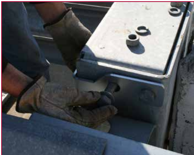
Securing Flush Mount Bracket
