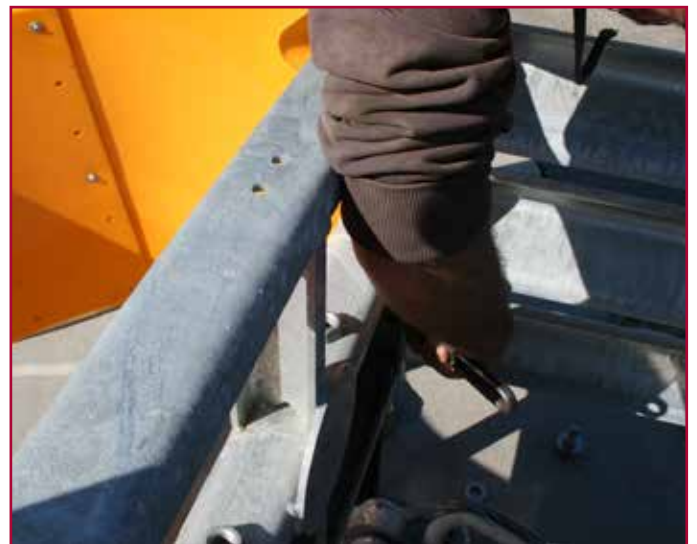
Installing One Side of Nose Cover
