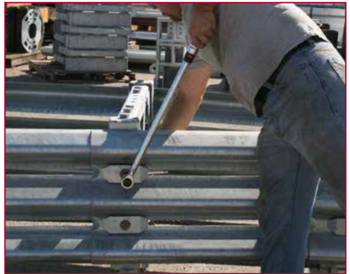
Applying Torque to Slider Bolts
