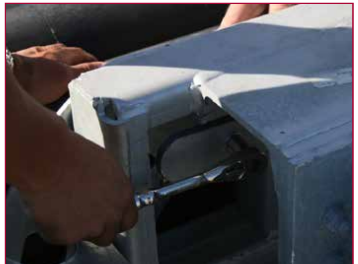
Bolting EAE to Compact Backstop
