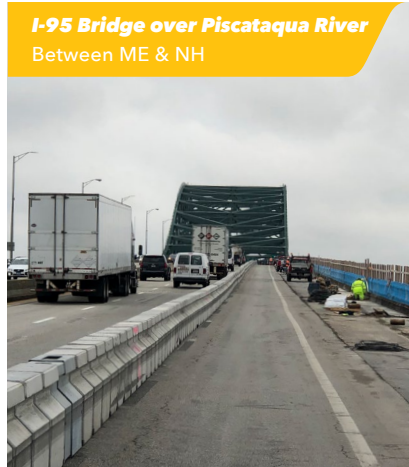
Safe & efficient expanded work zone during off-peak period (shoulder and middle lane rehab)
