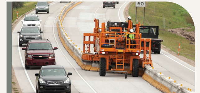
US 131 / GRAND RAPIDS, MI Pavement Rehabilitation: Four miles of Road Zipper System
