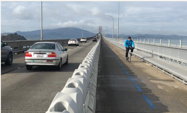
RTS Guard: A high performance, high containment barrier designed to separate bicycle and pedestrian paths from traffic.
