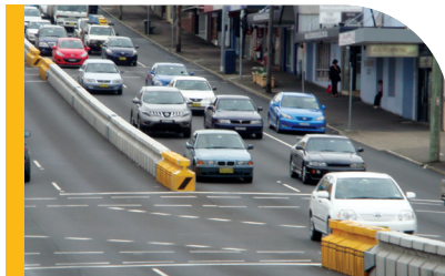
The Road Zipper system adds value by adding safety and efficiency on a limited Right-of-Way roadway. Moveable median application to add a 'Bus-Only' managed lane on a busy arterial street.
