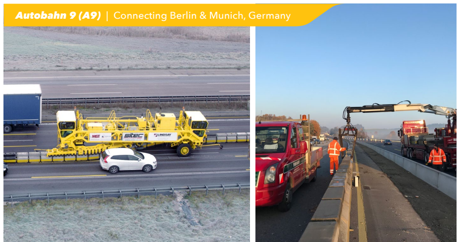
The moveable barrier provides more traffic lanes while offering the protection of positive concrete separation
