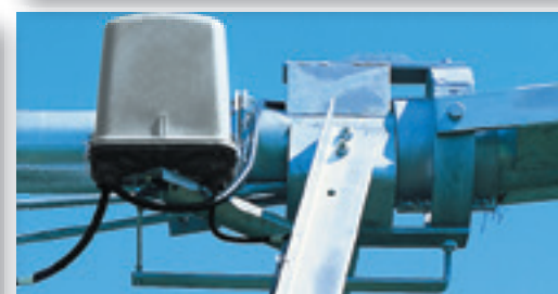
Uni-Knuckle span connector joint
